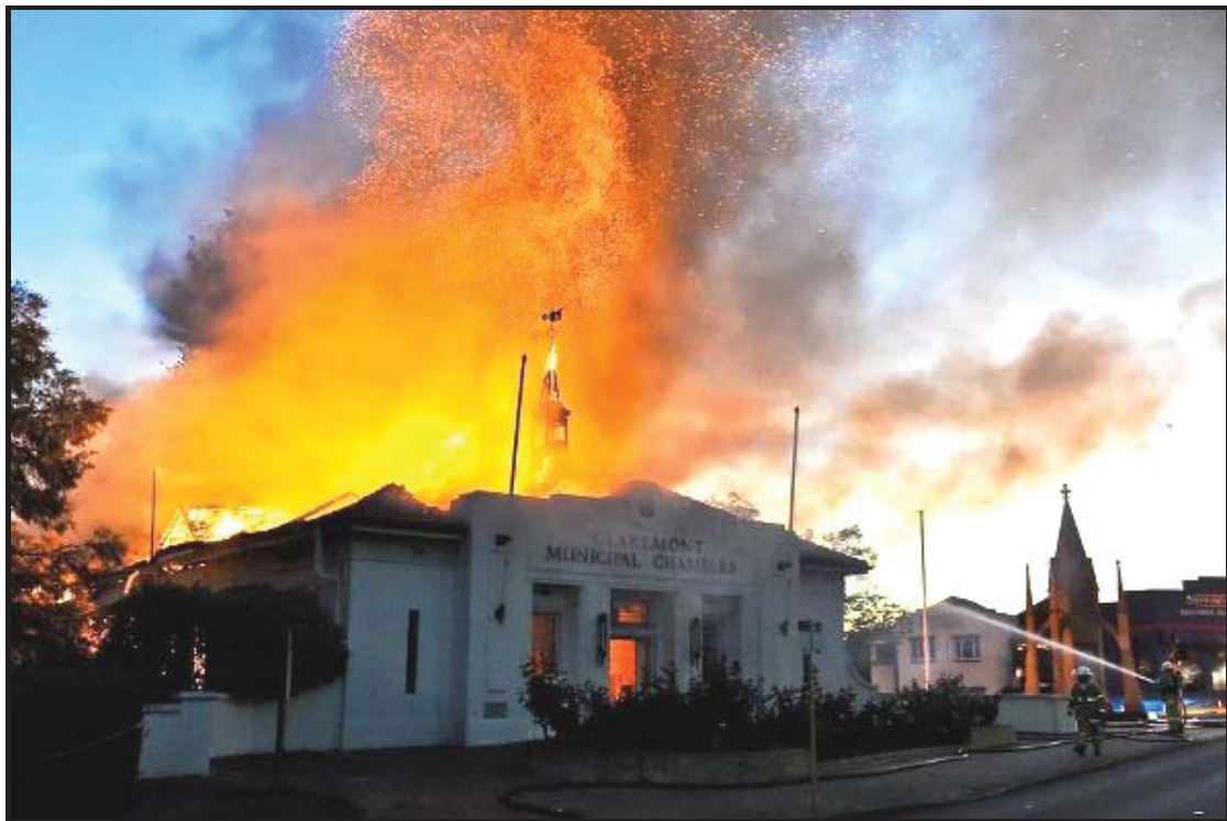
Fire at Town of Claremont Council offices 18 November 2010 (Photograph courtesy of Tom Vinnicombe)
